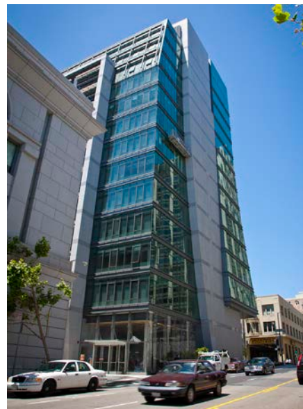
San Francisco Public Utilities Commission, San Francisco, CA
